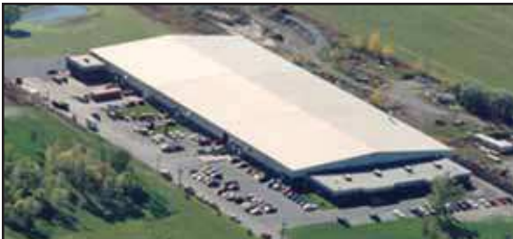
Parker Airtek Dryer Manufacturing Facility in New York State
