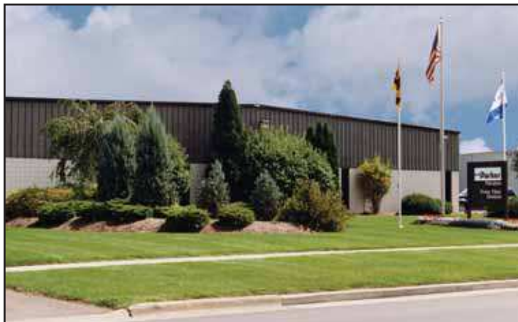
Parker Finite Filter Manufacturing Facility in Michigan
