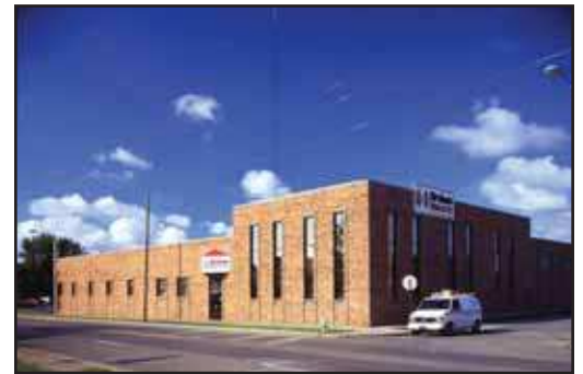
Brehob Electric and Crane & Hoist Division Headquarters in Indianapolis
