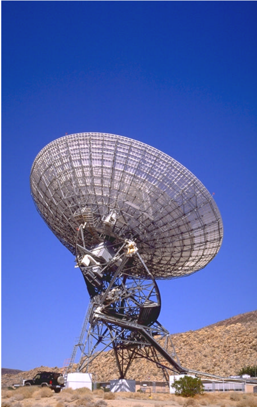
GAVRT ANTENNA AT NORTH LIMIT
