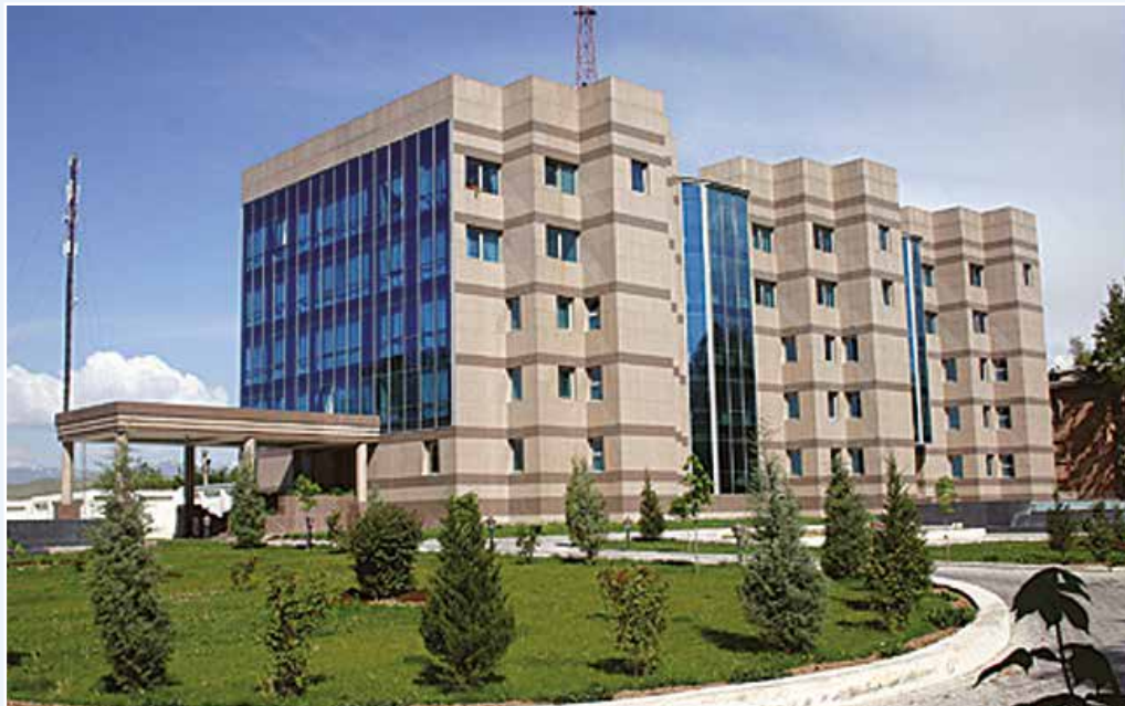
The National Bank of Tajikistan Administration building
