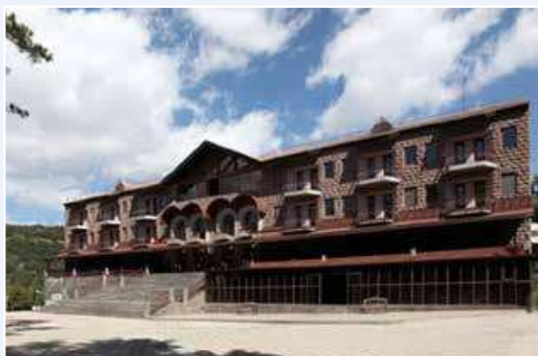
Training Centre of the Central Bank of the Republic of Armenia (Tsakhkadzor)
