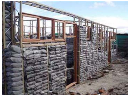
Figure 3: Construction of EcoBeam guest house
