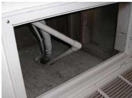
Pre-retrofit: Typical unsealed return plenum (left). Post-retrofit: Return plenum edges and seams are sealed, preventing return air from non-interior spaces, saves energy, and improves indoor air quality (right).
