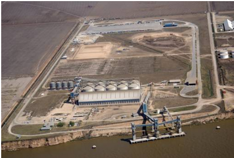
Figure 3: aerial view of the Noble port terminal
