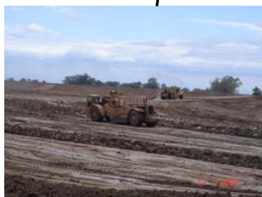
Plate 4: Northern Tailings Storage Facility establishment January 2005.
