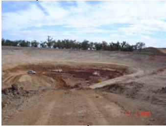
Plate 1: Crusher pit excavation – January 2005
