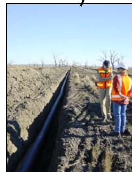
Plate 6: Pipeline trench across Lake Cowal.
