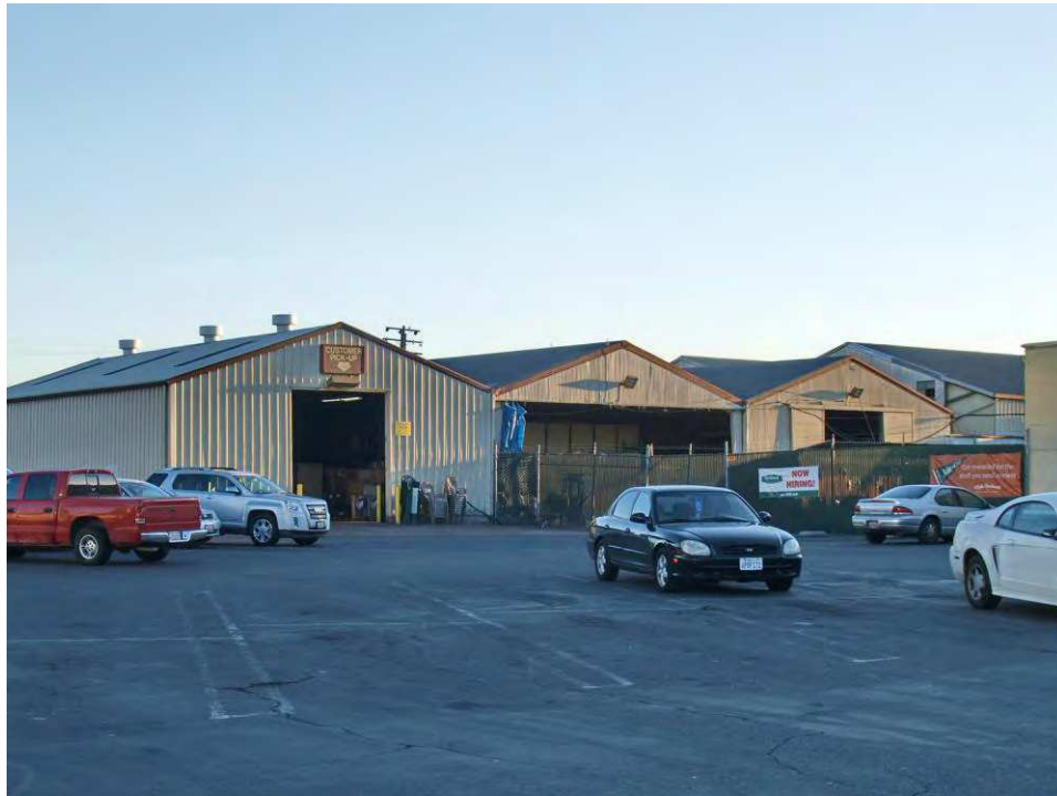
Warehouse and pick-up buildings to the south of retail store, viewed facing south.
