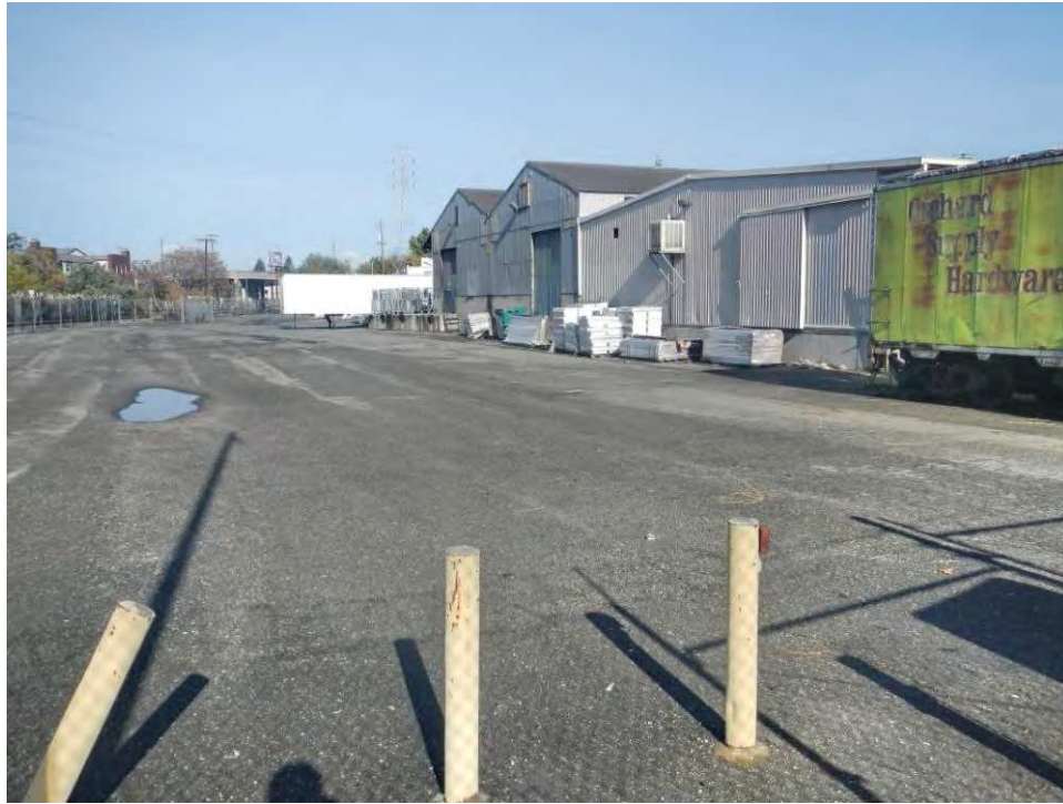
Rear railroad spur and docks at warehouse, viewed facing north from Auzerais Avenue.
