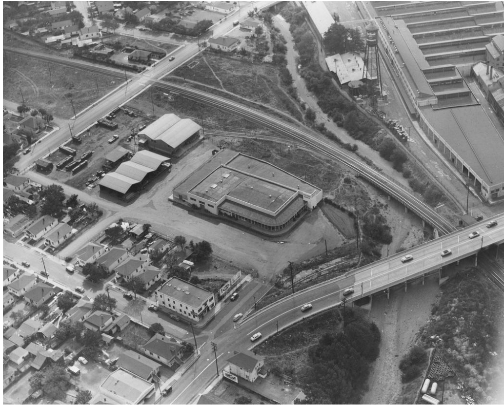
Aerial photo of 720 W. San Carlos site, ca. late 1940s. Courtesy of Orchard Supply Hardware.
