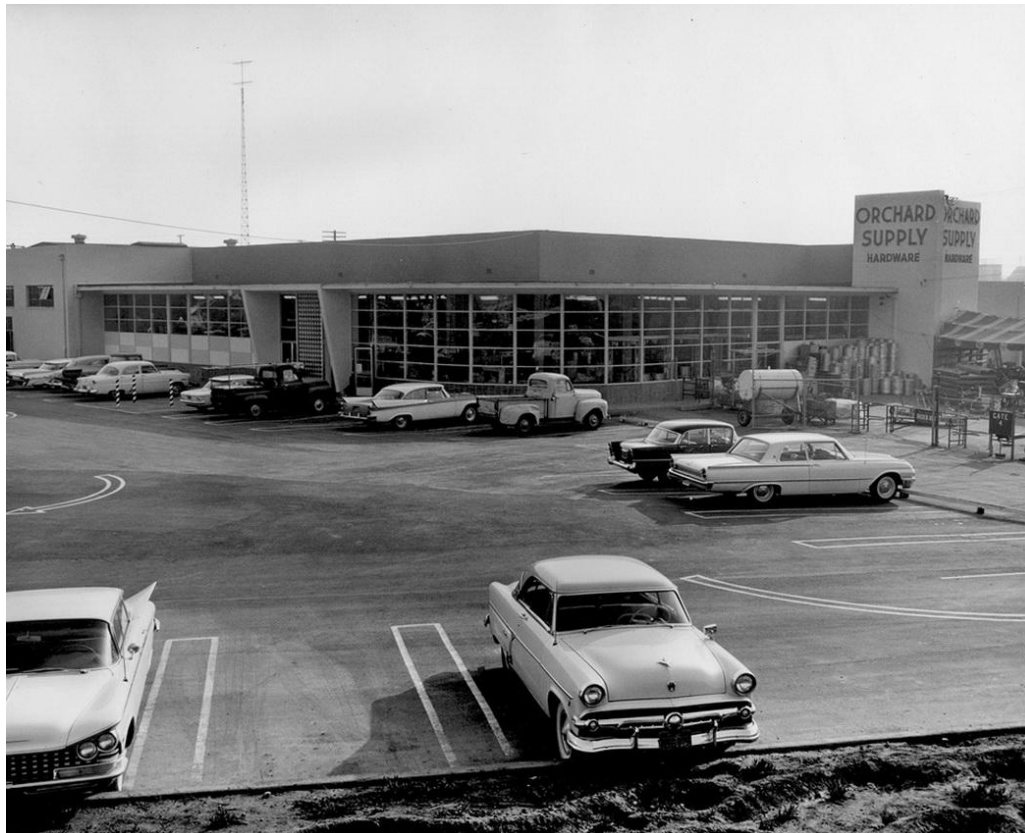
Photo of façade of 720 W. San Carlos St., ca. 1960. Courtesy of Orchard Supply Hardware.
