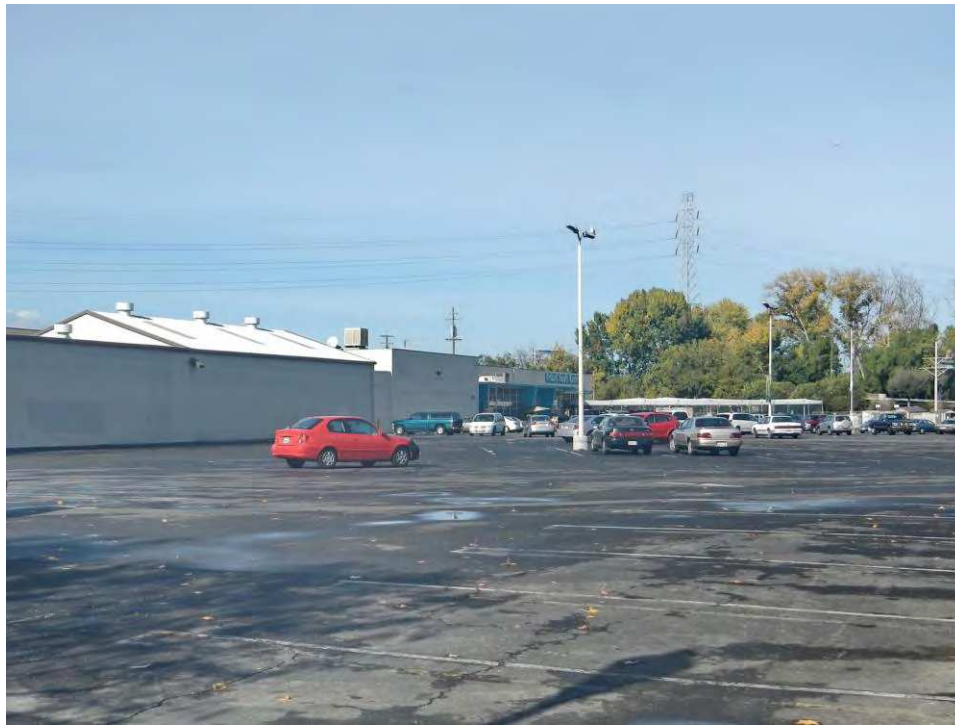
Overview of store entry from southeast.
