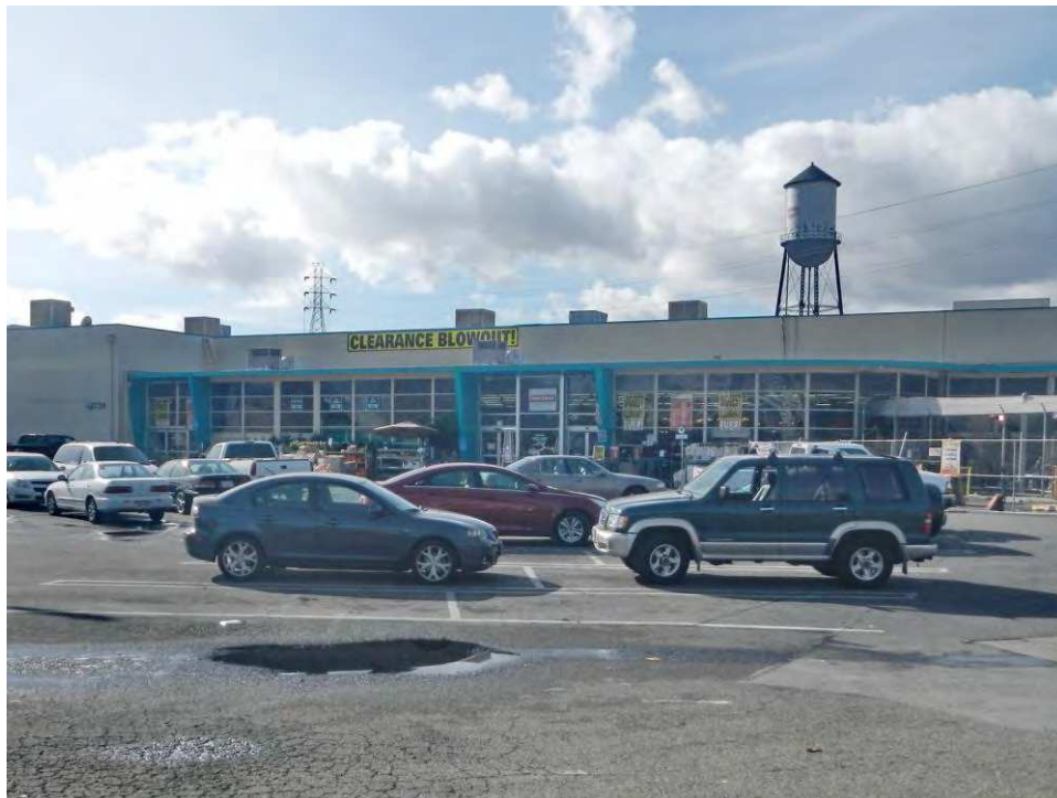
Left side of main entry façade viewed facing southwest.
