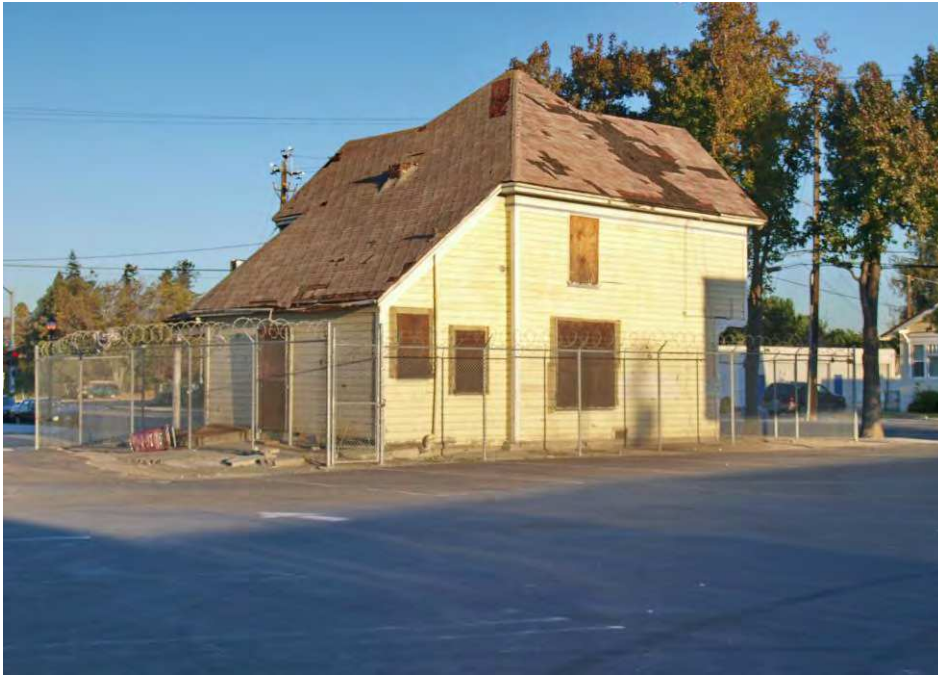
Rear elevation, viewed facing east from OSH parking lot.
