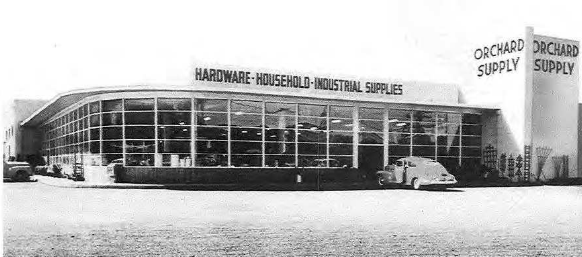
Façade of 720 W. San Carlos St., ca. late 1940s. Courtesy of Orchard Supply Hardware.
