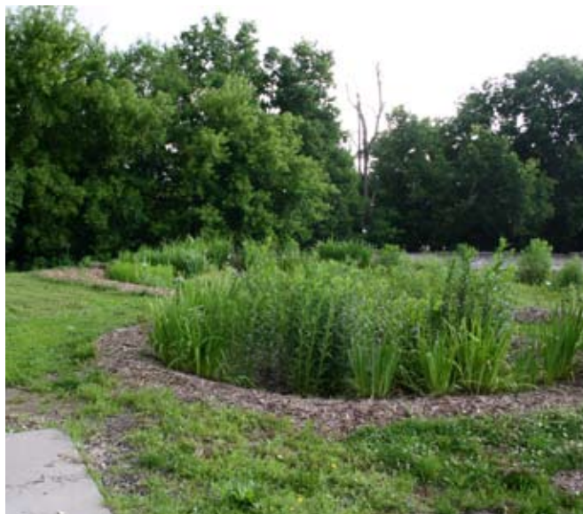
Above: This rain garden absorbs parking lot runoff at the Iowa Natural Resource Conservation Service office.
