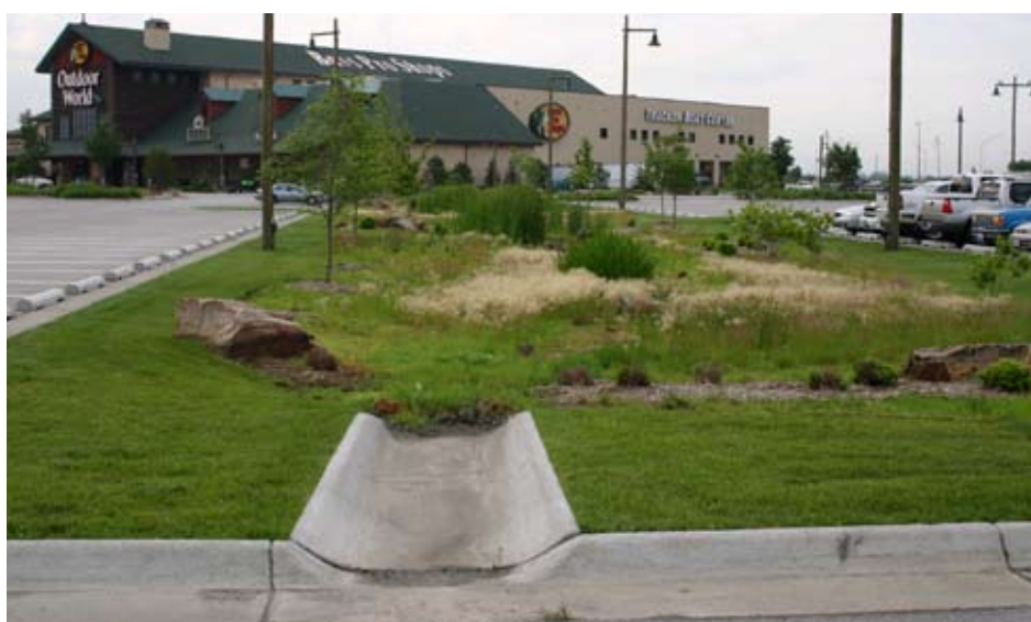
Below: Vegetated drainage swale between parking lots at Bass Pro Shops in Council Bluffs, Iowa. (Photos courtesy Steve Rodie)
