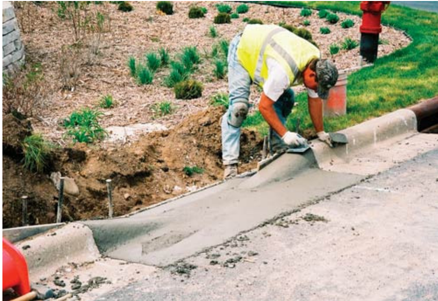
Cuts in the curb allow stormwater to enter the gardens from the street.
