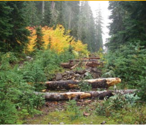
As part of our restoration on the Upper Kachess Road pictured here, adding big logs as woody debris helps restore an old road bed. Photo William C Ehinger/USFS
