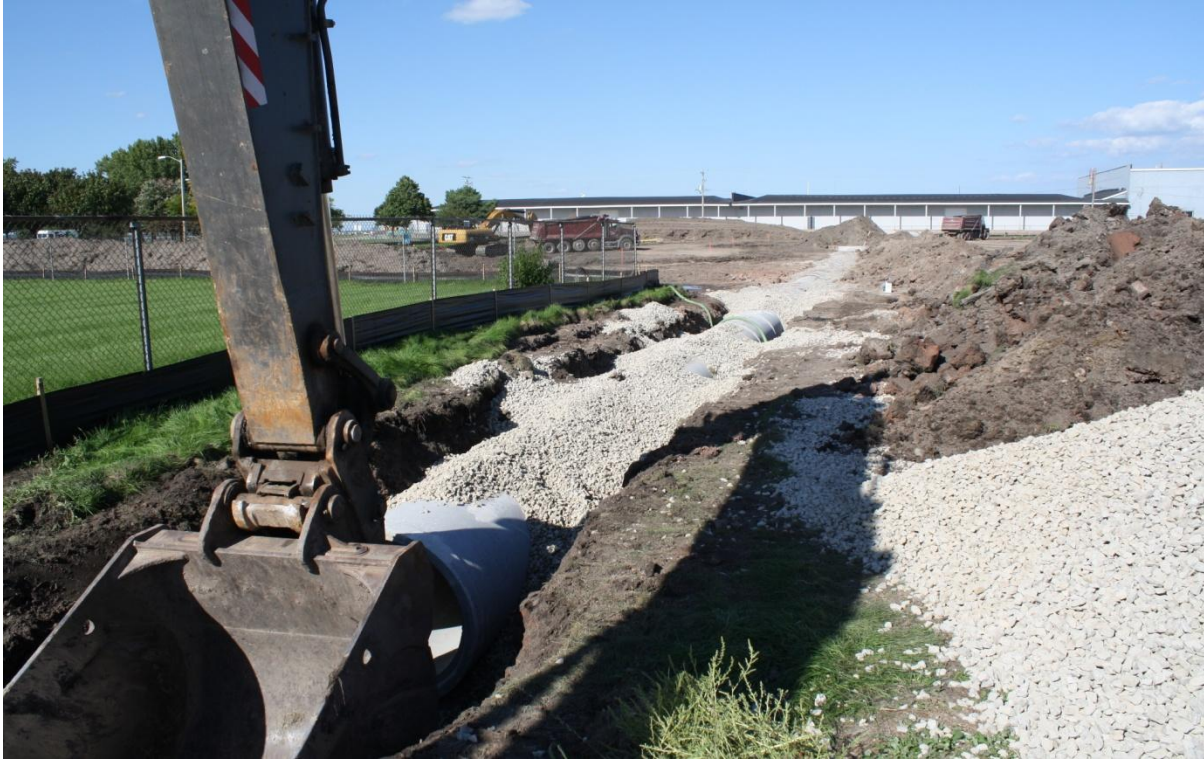
Stormwater piping looking west to detention pond.
