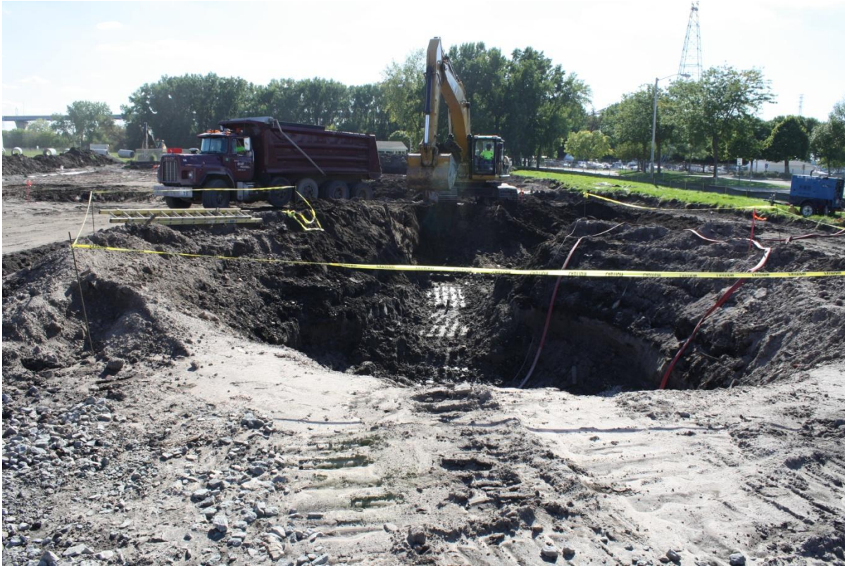
Stormwater detention pond excavation looking south.
