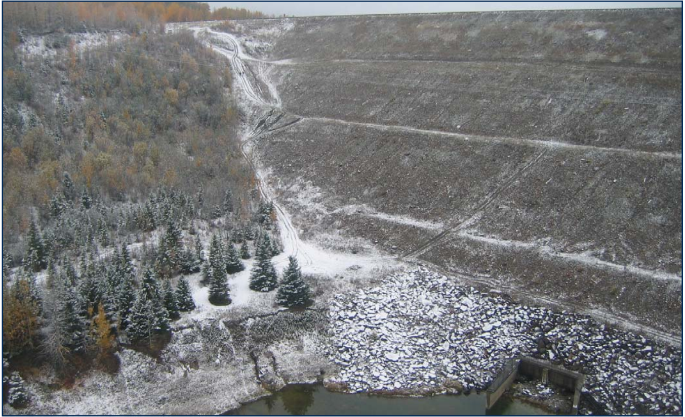
Deep erosion channels are part of the damage caused by all terrain vehicles at the Brazeau dam site.
