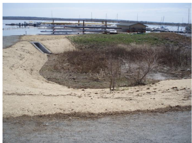
Photo 9 Reconstructed Water Quality Basin
