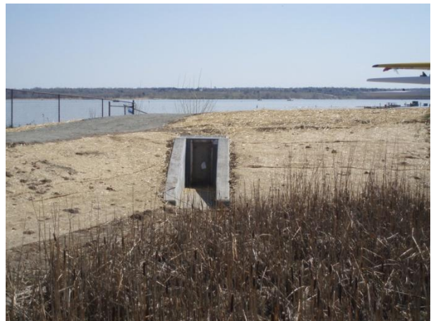
Photo 8 Reconstructed Water Quality Basin
