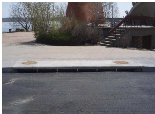
Photo 4 Constructed 15-Foot Inlet
