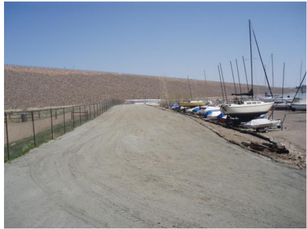
Photo 6 Constructed Overflow Storage Parking Area
