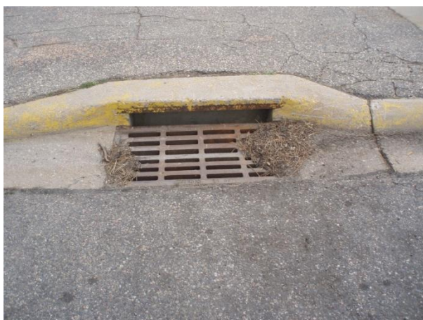
Photo 3 Existing 5-Foot Inlet
