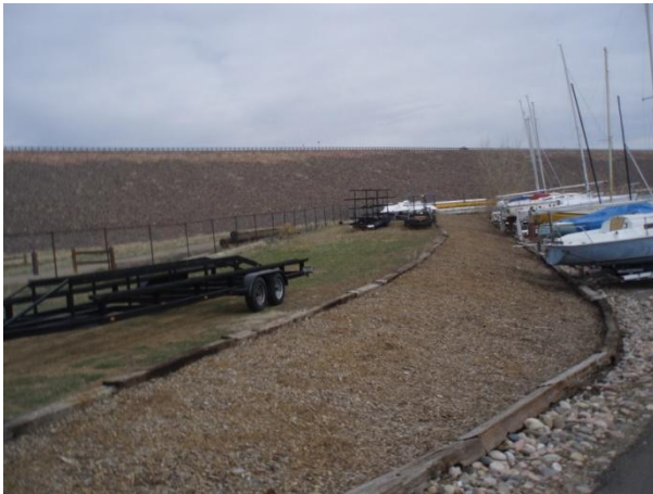
Photo 5 Existing Overflow Storage Parking Area
