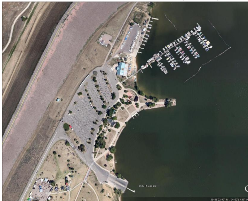
Photo 1 West Boat Ramp Parking Lot @ Cherry Creek Reservoir
