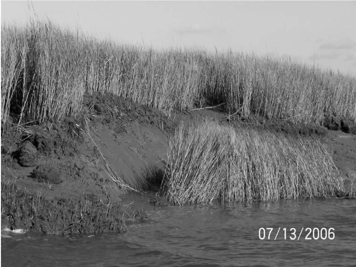
Figure 58: Photo of large masses of marsh slumping. This photo was taken in the area between stations 16 and station 18.
