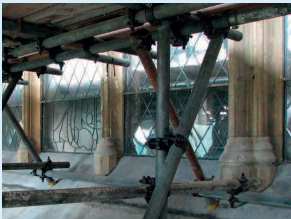
Trial installation of protective glazing designs on the East Window of York Minster, which were shown on an excursion during the master class
