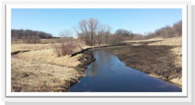
Early April CRWD PO 6 Project Enhancement | Looking north from HWY 55, addition of channel to reduce phosphorus load to Cedar (original stream to the left)
