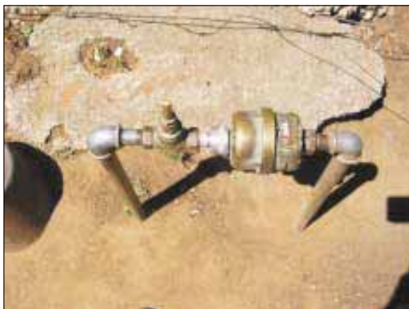
Figure 6: Typical Domestic Consumer Meter Installations in South Africa
