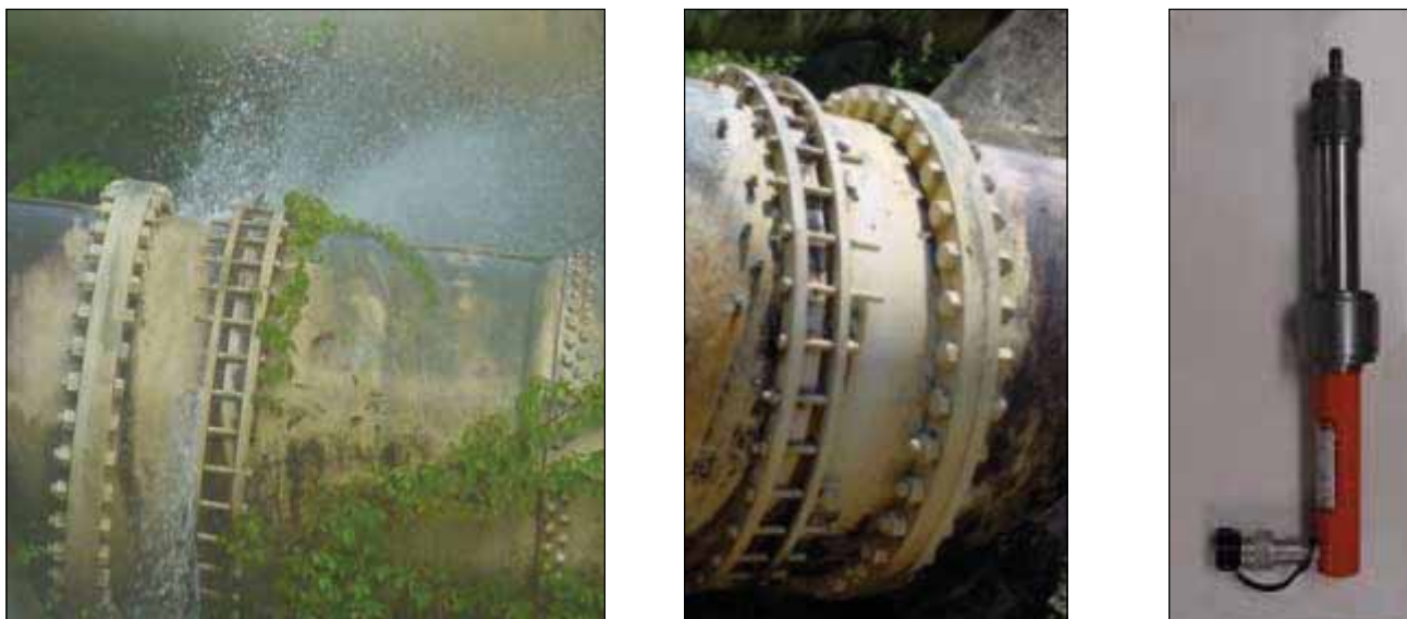
Figure B-3: Repair of leaking expansion joint (Courtesy Coltonline website)
