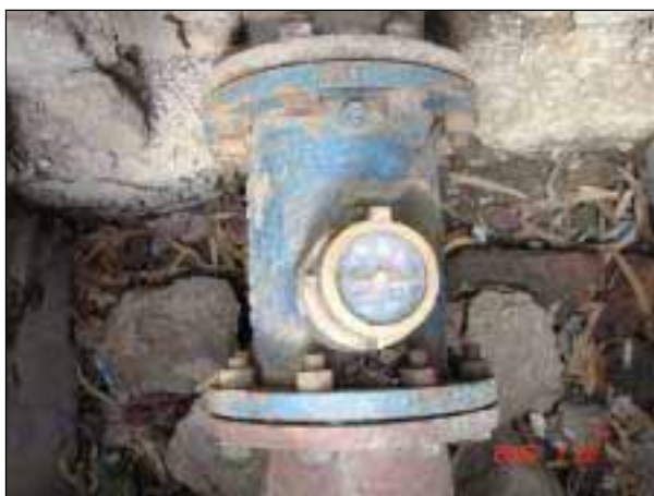
Figure 4: Typical Bulk Consumer Meters in Indore (Continue)
