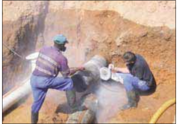
Figure C-2: a) Exposed pipe with temporary supports b) Cutting into asbestos cement pipes
