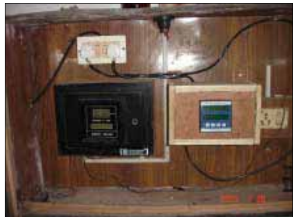
Figure 3: Typical Bulk Consumer Meters in Indore
