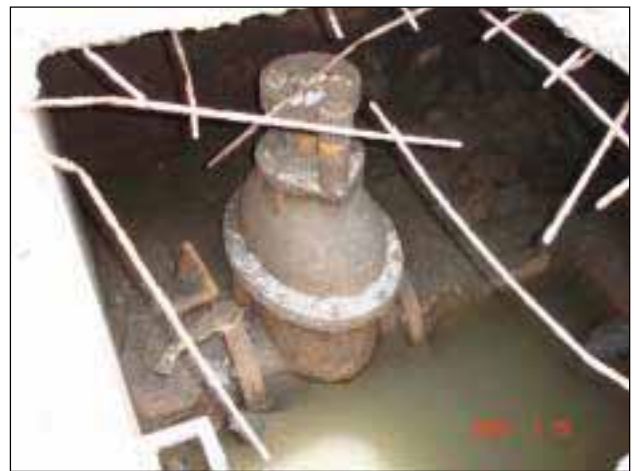
Figure 11: Typical Leaking Valves throughout Indore
