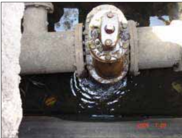
Figure 11: Typical Leaking Valves throughout Indore
