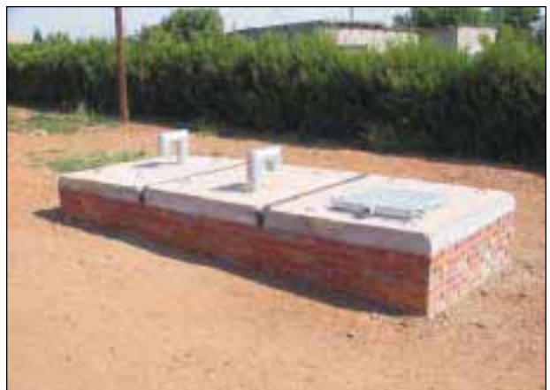
Figure C-4: a) Brickwork completed with anchor block visible b) Completed chamber with lockable manhole cover
