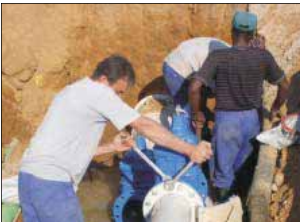
Figure C-3: a) Installing new pipework and fittings b) New pipework completed with concrete floor in place
