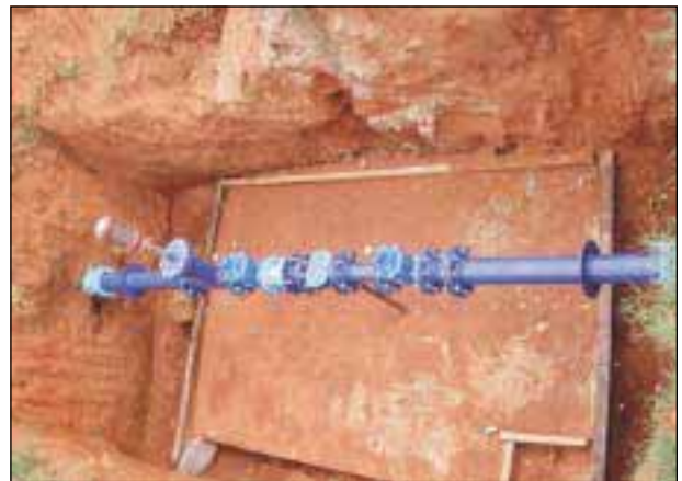
Figure C-3: a) Installing new pipework and fittings b) New pipework completed with concrete floor in place
