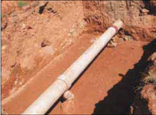
Figure C-2: a) Exposed pipe with temporary supports b) Cutting into asbestos cement pipes
