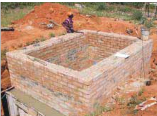
Figure C-4: a) Brickwork completed with anchor block visible b) Completed chamber with lockable manhole cover
