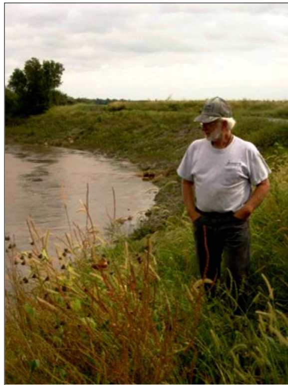
David Royer, above, surveys the streambank stabilization work done on the Delaware River on his farm. Photo by C. Pantle
