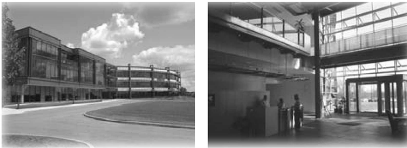
Figure 2. Wing Construction and Atrium.
