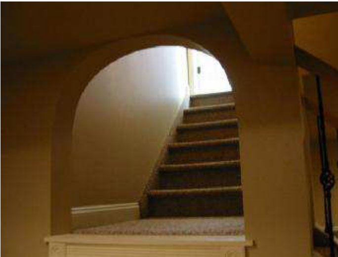
Install balusters at open arch at basement stairway landing.
