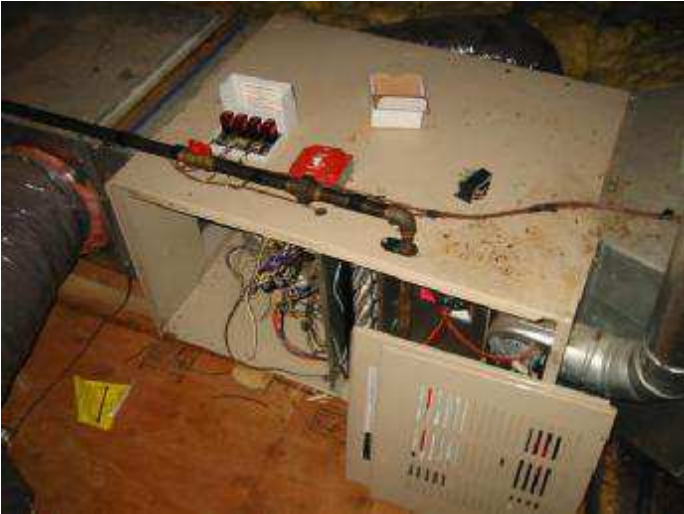
Furnace in attic under repair.
