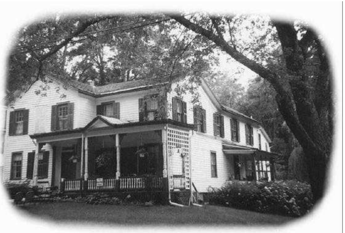
177 Union Street, Sharon Springs The Brustman House as it looks in 2000, essentially the same as in 1944.
