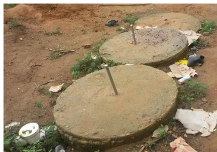
Figure 10: Septic Tank in Barracão dos Mendes (Image taken by the author)
