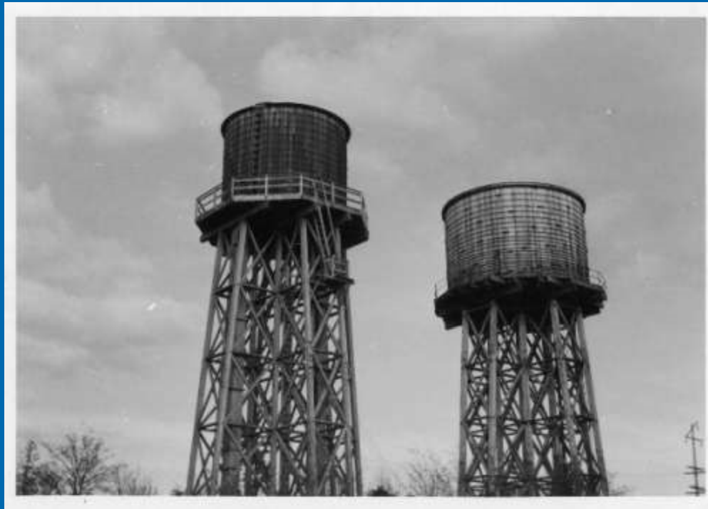
Water Towers, 1951-1970, Water District No. 54 Located on the north side of the Des Moines Field House, near the current skateboard park
