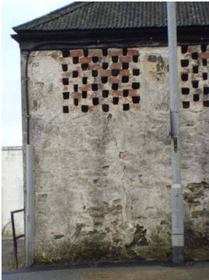
The north gable of the short return of the drying shed indicating cracking and repointing in gable wall
