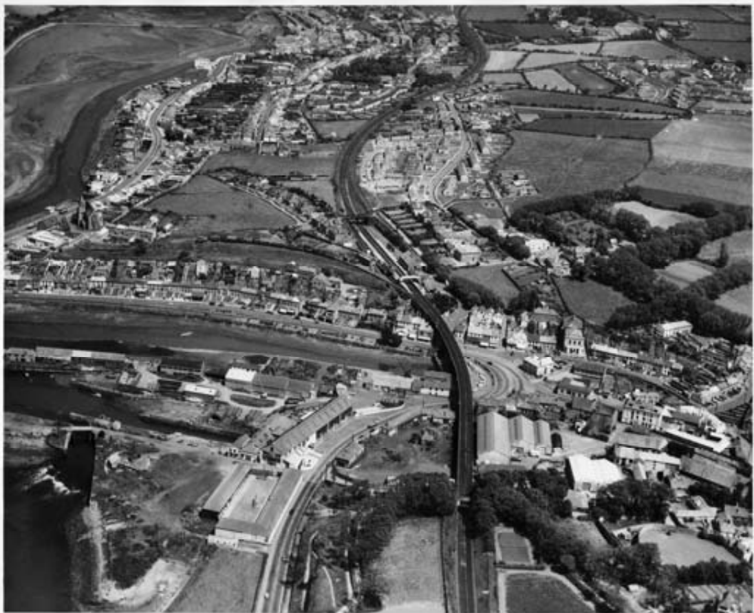
Aerial photograph of the site from the west in thy 1960's with the lime kilns still visible Above 2 No. photographs reproduced by consent from Hayle Community Archive
