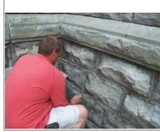
and new caulking has been applied. A special tuck-pointing tool was designed to apply a "grapevine joint" that will give the mortar a vine like appearance in the middle of the mortar.
