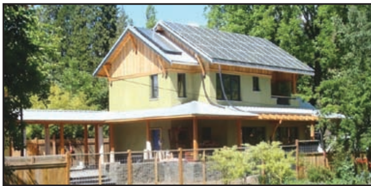
Eugene's first Passive House has it all—from solar energy and salvaged materials, to organic gardens and chickens—on a surprisingly small footprint. It's one house you won't want to miss.
