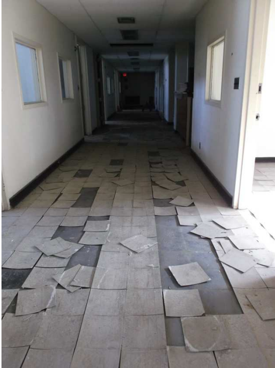
Floor Tiles Lifting in Corridor
