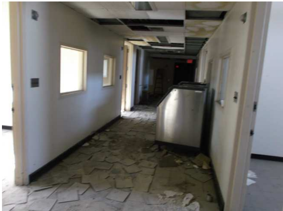
Floor Tiles Lifting in Corridor
