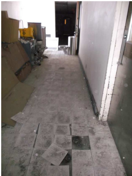
Floor Tiles Lifting in Corridor (Typ.)
