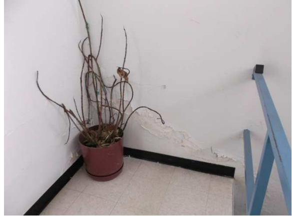
Water Infiltration In Stairwell
