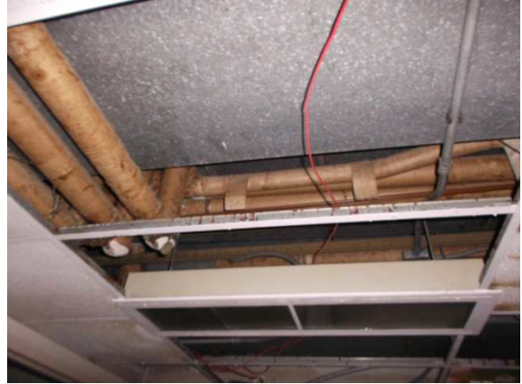
Wrapped Piping in Cooridor Ceiling
