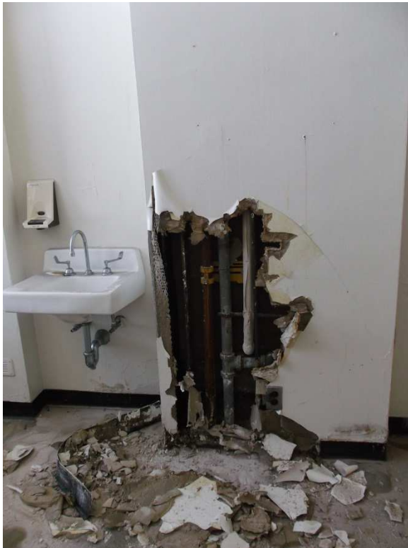
Section of Wall Removed to Fix Leak
