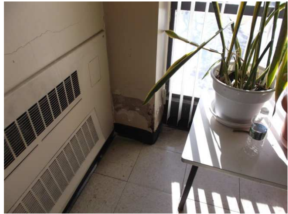
Water Infiltration Second Floor
