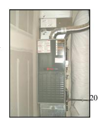
The damper located in the main air duct next to the furnace (if applicable) is also a good tool to maintain peak heating and cooling efficiency. The air duct transfers air to the second floor and the damper within allows the homeowner to seasonally regulate the flow of cool and warm air.
