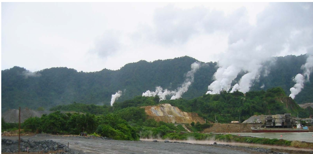
Figure A2: Steam Being Vented to Atmosphere as a Component of Current Mining Operations
