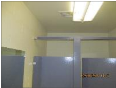
Photo 12 – Drywall ceiling in Boys 109.
