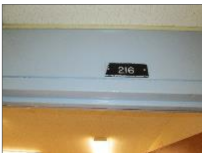
Photo 16 – Typical view of drywall above doorframes found only on doorways common to corridors.
