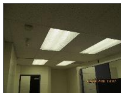
Photo 10 – Non-asbestos ceiling tile in Boys WR 120 and 120V.
