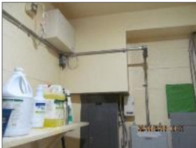
Photo 14 – Drywall on wall of Custodian 208.
