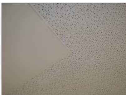
Photo 11 - Example of non-asbestos 12" x 12" glued-on ceiling tile.
