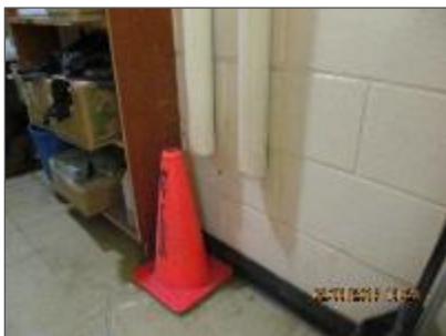
Photo 5 – Seams and butt ends of fibreglass insulation with parging cement on domestic water pipes in Custodian 100B.
