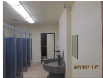
Photo 13 – Drywall ceiling in Girls WR 114.
