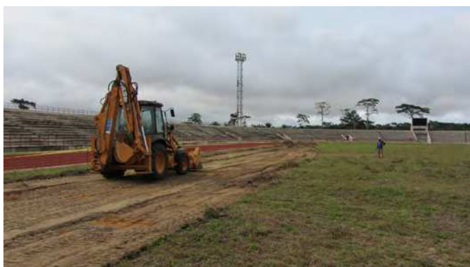
Figure 4: Vegetation and first soil layer removal.
