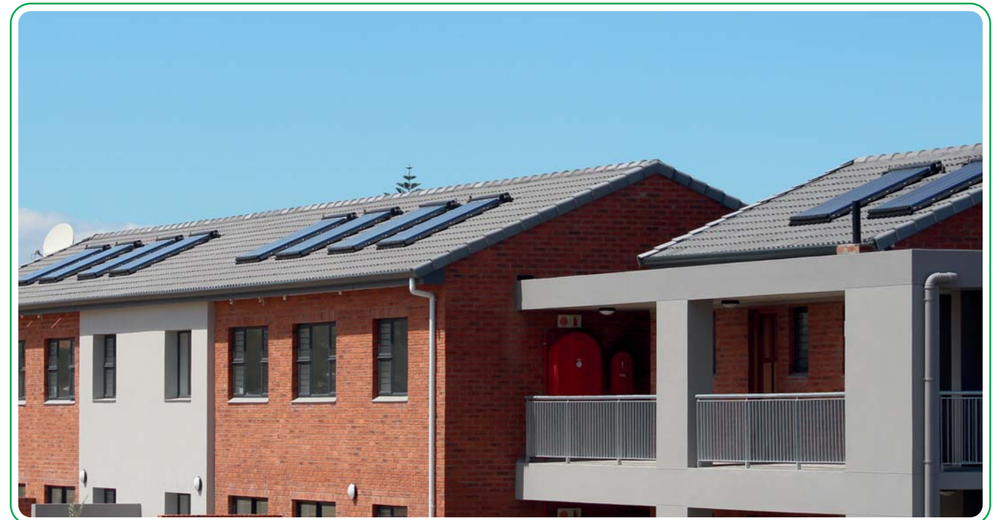
Solar geysers being installed at Bothasig Gardens
