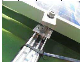
P-04: Solar module earthing device (if required) – how panel is earthed to rail
