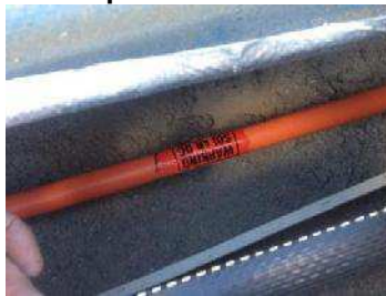
P-09: DC cable identification, mechanical protection and reticulation
