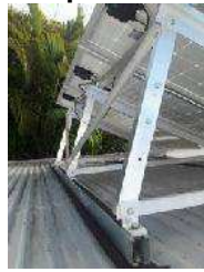
P-04: Solar module earthing device (if required) – how panel is earthed to rail
