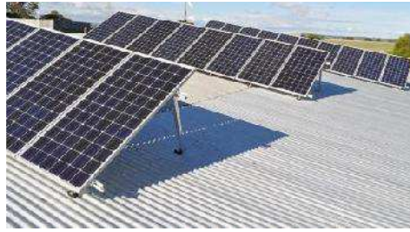
P-03: Roof fixing brackets securing rails in position / fixing of brackets to roof.
