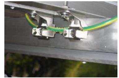
P-05: Solar module earthing device (if required) – how earth cable is secured (note Gal Spray)
