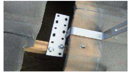
P-04: Solar module earthing device (if required) – how panel is earthed to rail
