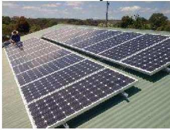
P-03: Roof fixing brackets securing rails in position / fixing of brackets to roof.
