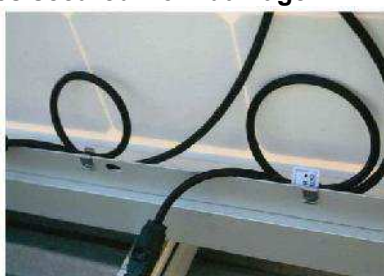
P-10: Under-module cabling / cables secured from damage
