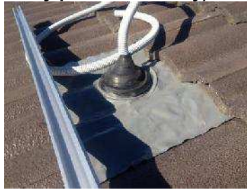
P-08: Roof penetration (main cable entry point from array)
