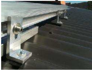
P-04: Solar module earthing device (if required) – how panel is earthed to rail
