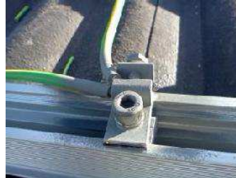
P-06: Rail joiner / Splice kit (showing continuity between segments)
