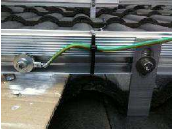
P-06: Rail joiner / Splice kit (showing continuity between segments)
