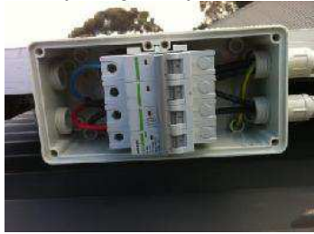
P-07: Rooftop isolator and string fuses (if required)
