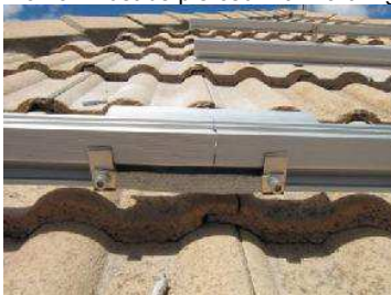
P-06: Rail joiner / Splice kit (showing continuity between segments)
