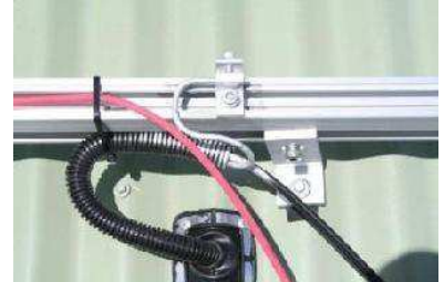
P-05: Solar module earthing device (if required) – how earth cable is secured (note Gal Spray)
