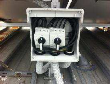
P-08: Roof penetration (main cable entry point from array)
