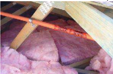
P-09: DC cable identification, mechanical protection and reticulation
