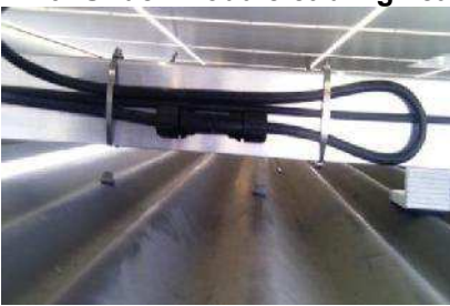
P-10: Under-module cabling / cables secured from damage
