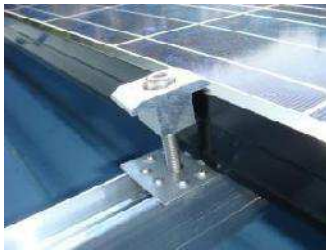
P-04: Solar module earthing device (if required) – how panel is earthed to rail
