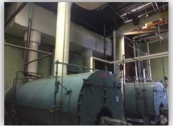
created by installing a steam to hot water heat exchanger in the boiler room. Hot water was created from the steam and was pumped to the ancillary heating equipment located in the new section. For the most part, the hot water system uses a DMS pneumatic overlay to adjust the temperature set points of the system.
