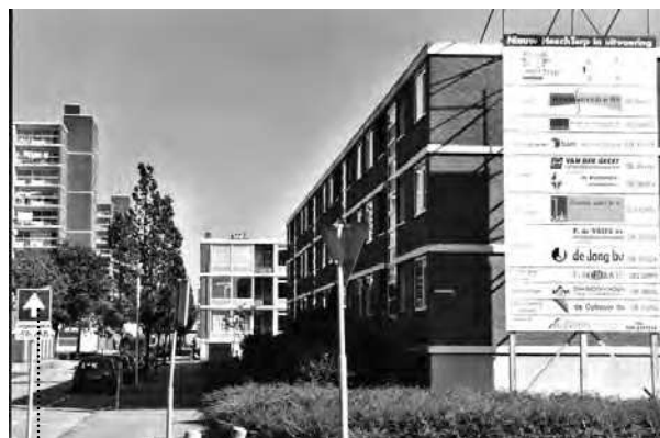
Figure 6. Refurbishment of low rise flats.
