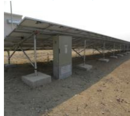
Figure 2.7: Spread footing
