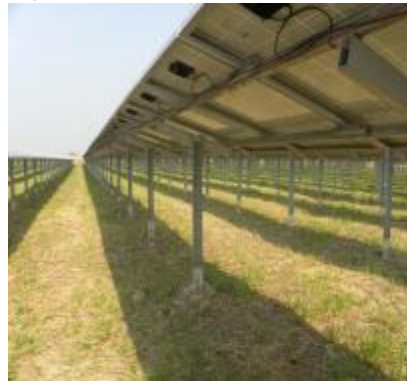
Figure 2.6: Piled foundation
