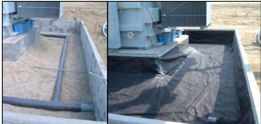
Transformer Pad (Before / After)
