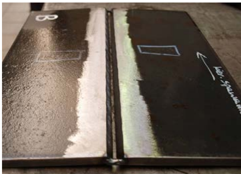
Fig. 3. Weld groove with small amount of anti-spatter substance after making tack welds
