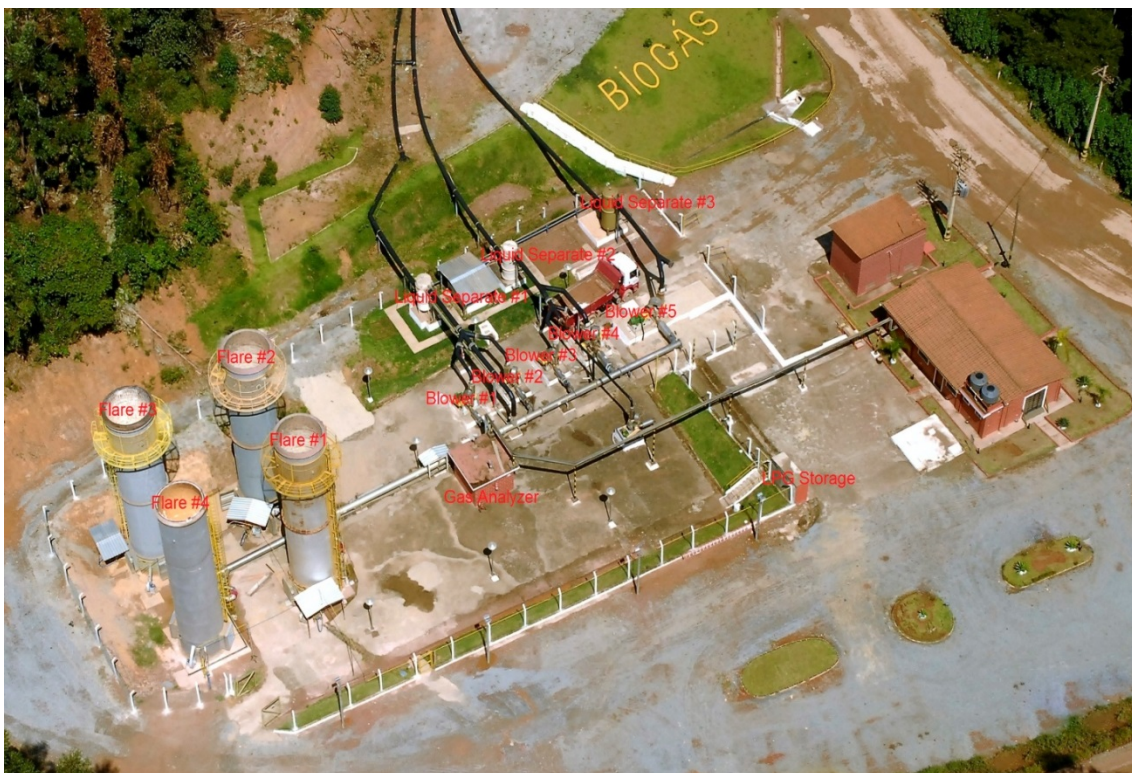
Figure 3 – Aerial view of the project’s LFG destruction plant (picture dated April 2013).
