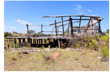
Image 31: Remaining framework and piers. Facing south. File-6789.
