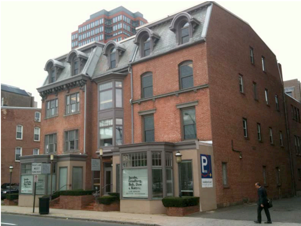
2. Northeast view from Orange Street, camera facing southwest
