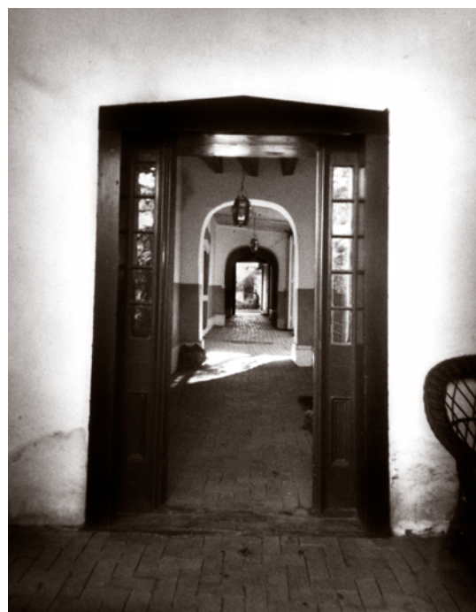
This undated photograph by Laura Gilpin was used to determine the height of the micacious clay band in the zaguán.
