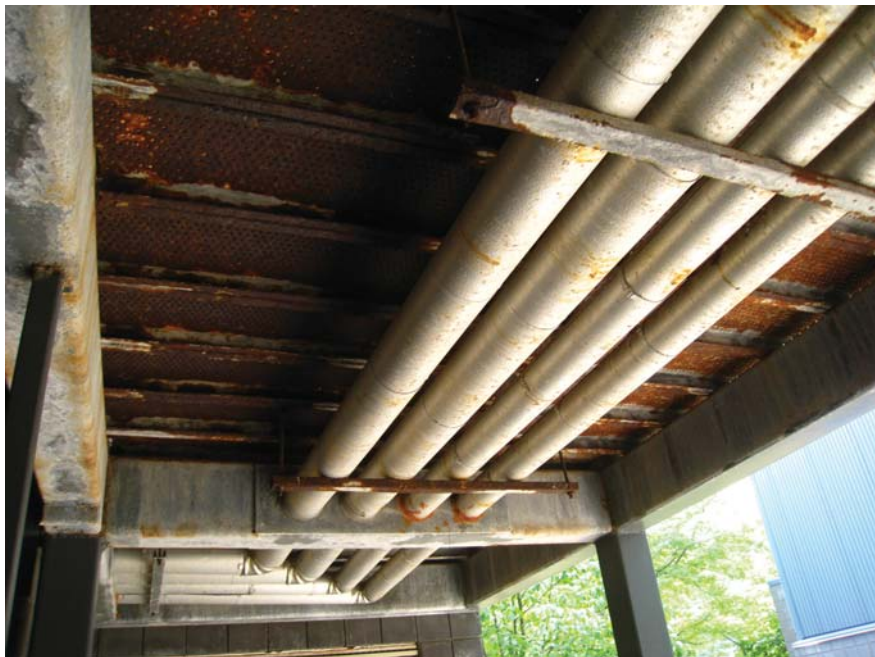
Photo 1: Underside of second floor access deck
