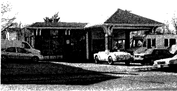
Gas Station 6300 Block of Arsenal
