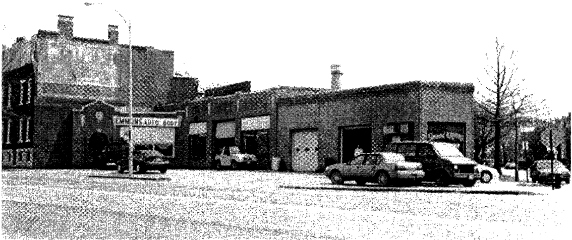
Service Garage 2230 Gravois
