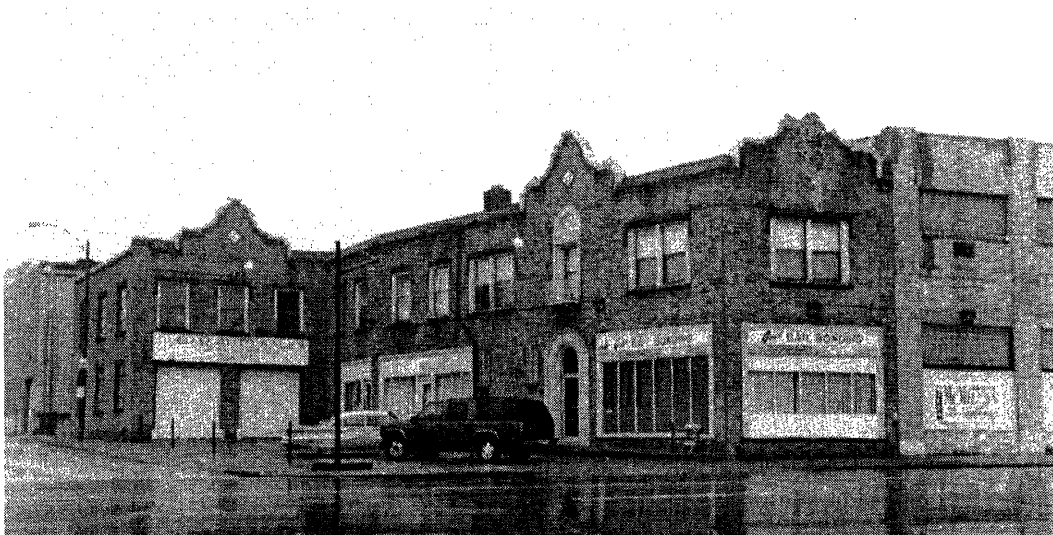
Becker-Lehman Sales Company Building, (Tire Company) 3043 Olive
