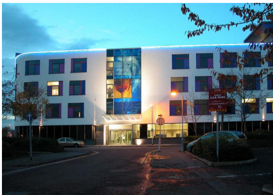
Hollywood Arches Community Health Centre, Northern Ireland
