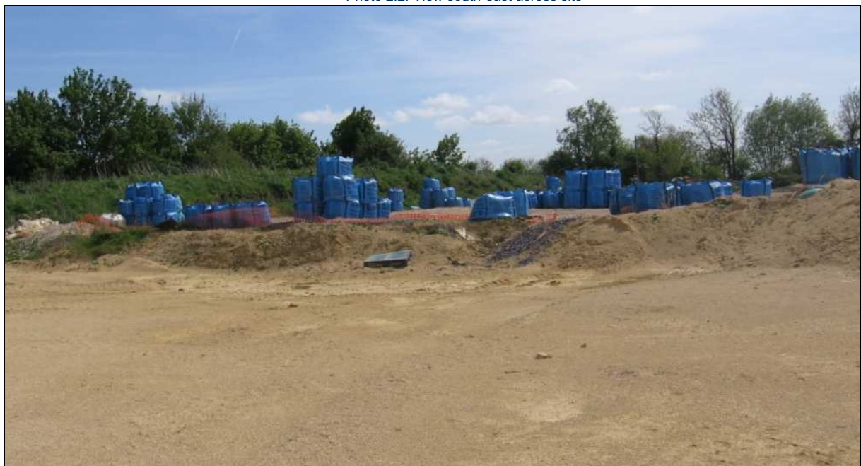
Photo 2.2: View south-east across site
