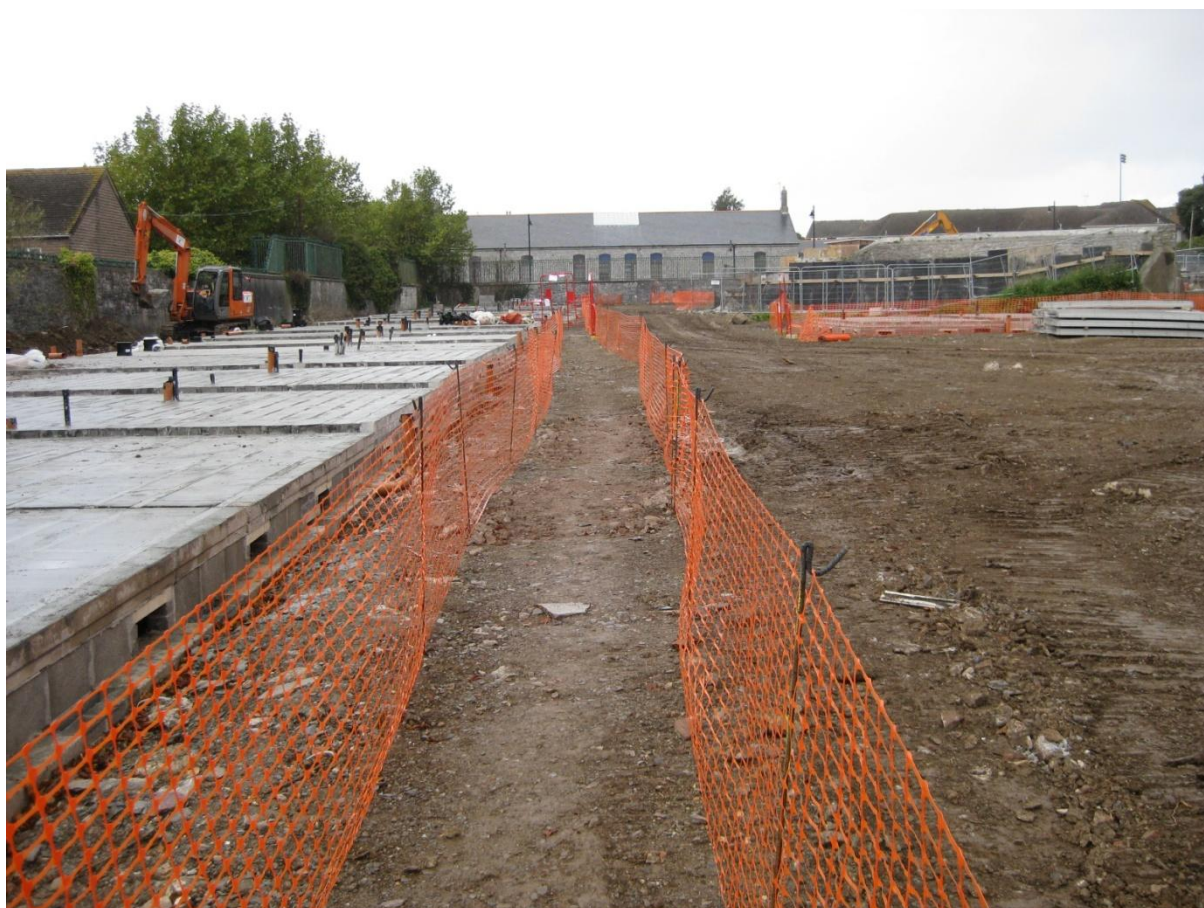
Well installed orange netting demarking pedestrian walkway from mobile plant areas
