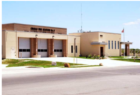
City of Cibolo Fire Station 2
