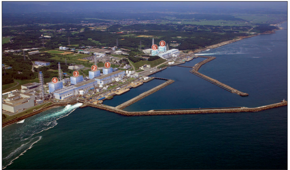
Fig. 2. Aerial photo of the Fukushima Daiichi nuclear power plant before March 11, 2011.
